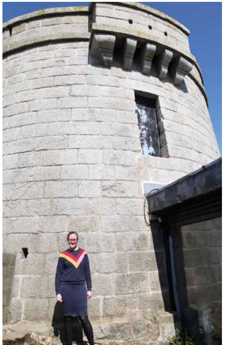
View of the Tower showing the original entrance on the first floor.
