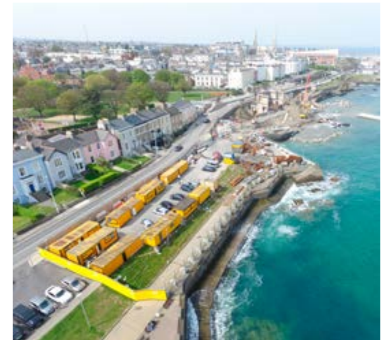
Dún Laoghaire Baths Construction Site
